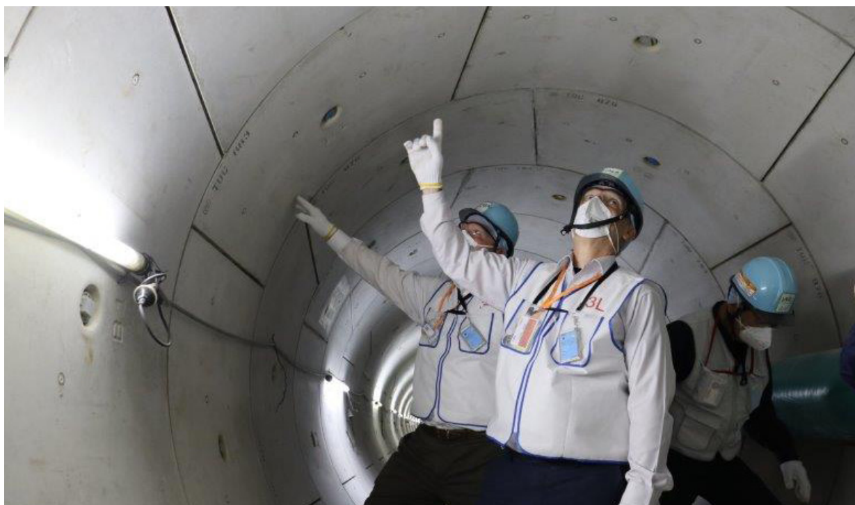
Figure 3.8. Pre-service inspection of ALPS discharge facility
